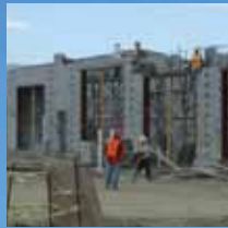
Recycled concrete used throughout
