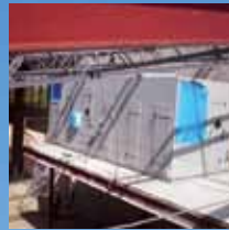
Water cascade direct/indirect evaporative cooling and high energy efficiency HVAC system
